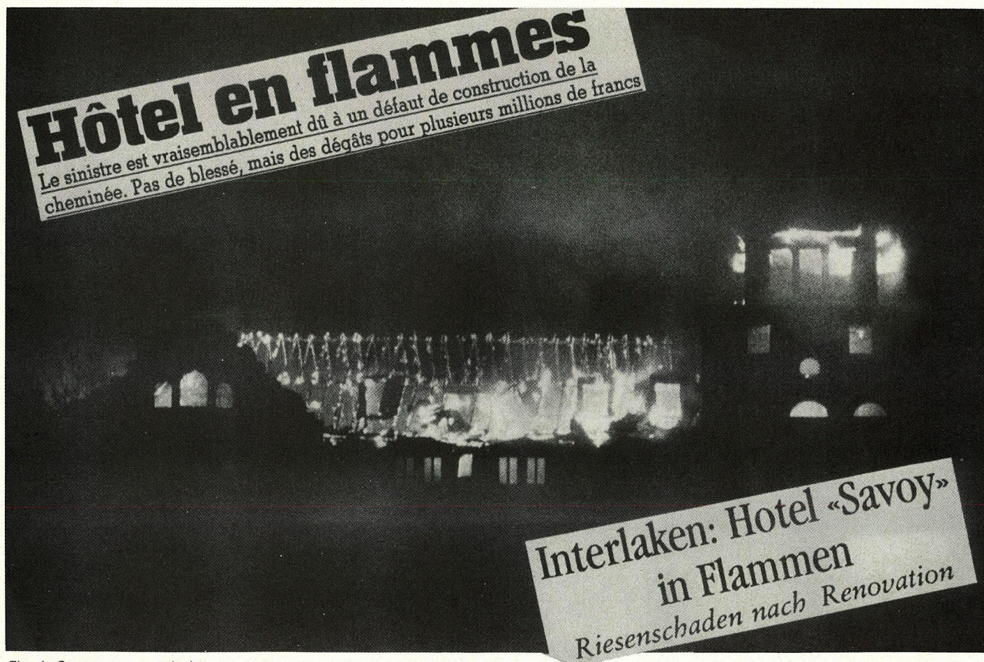
Fig. 1. Sans commentaire! This fire was probably due to a lack in the construction of the chimneypiece.
